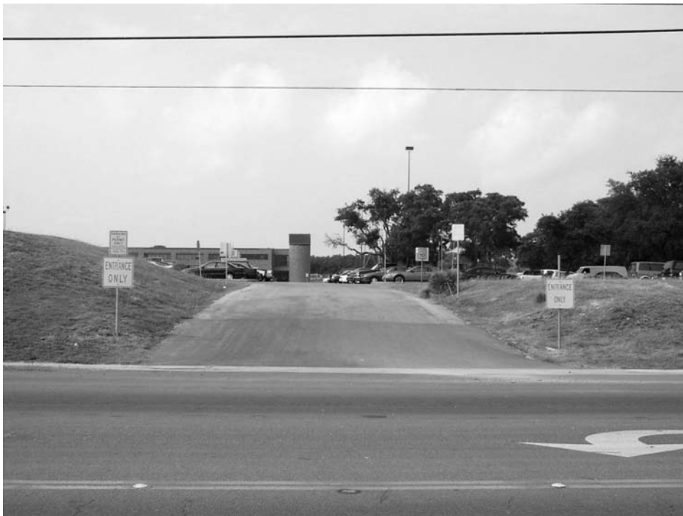
Figure 7-224. Driveway 2 (Facing Southwest).
