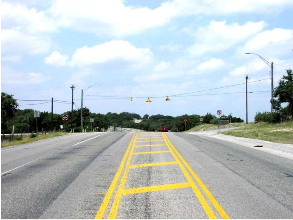
Figure 7-189. Driveway 1 (Facing West).
