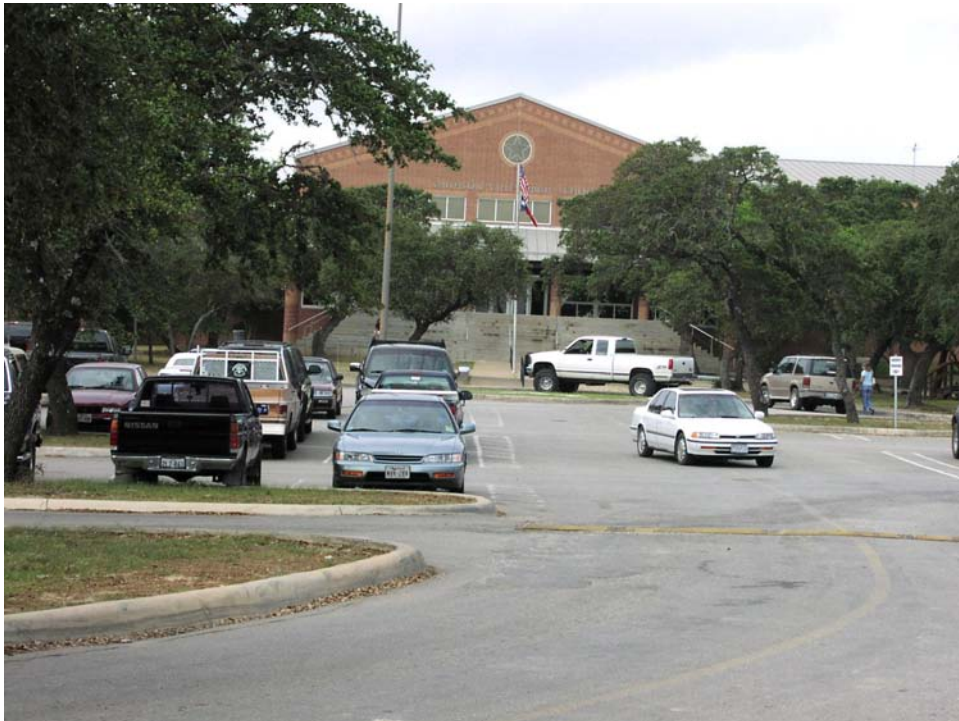
Figure 7-203. Parent Drop-Off/Pick-Up Zone and Employee Parking Lot (Facing South).
