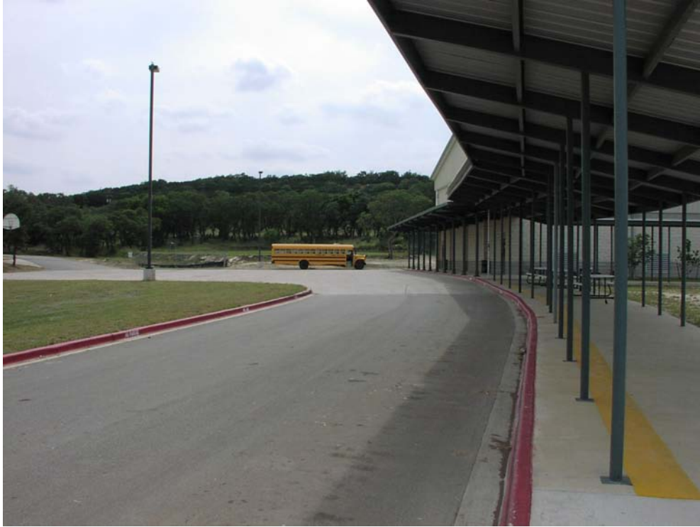
Figure 7-113. The Middle School Bus Drop-Off/Pick-Up Zone (Facing West).
