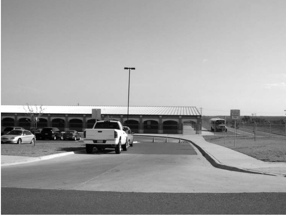
Figure 7-73. Driveway 2 (Facing North).
