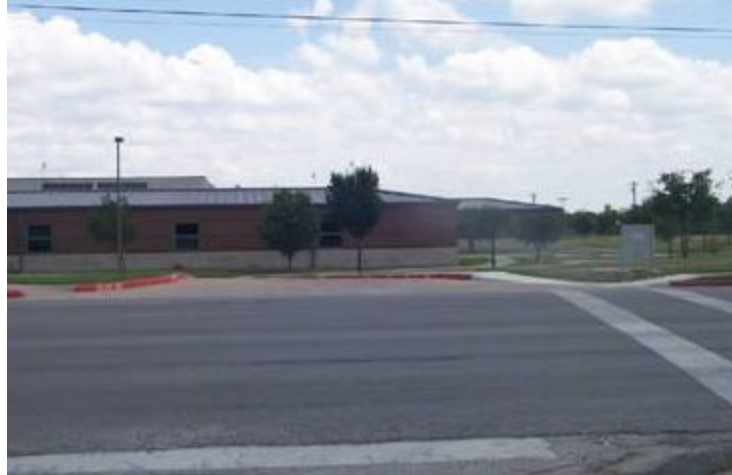
Figure 7-157. Entrance Driveway to the Visitor Semicircle.
