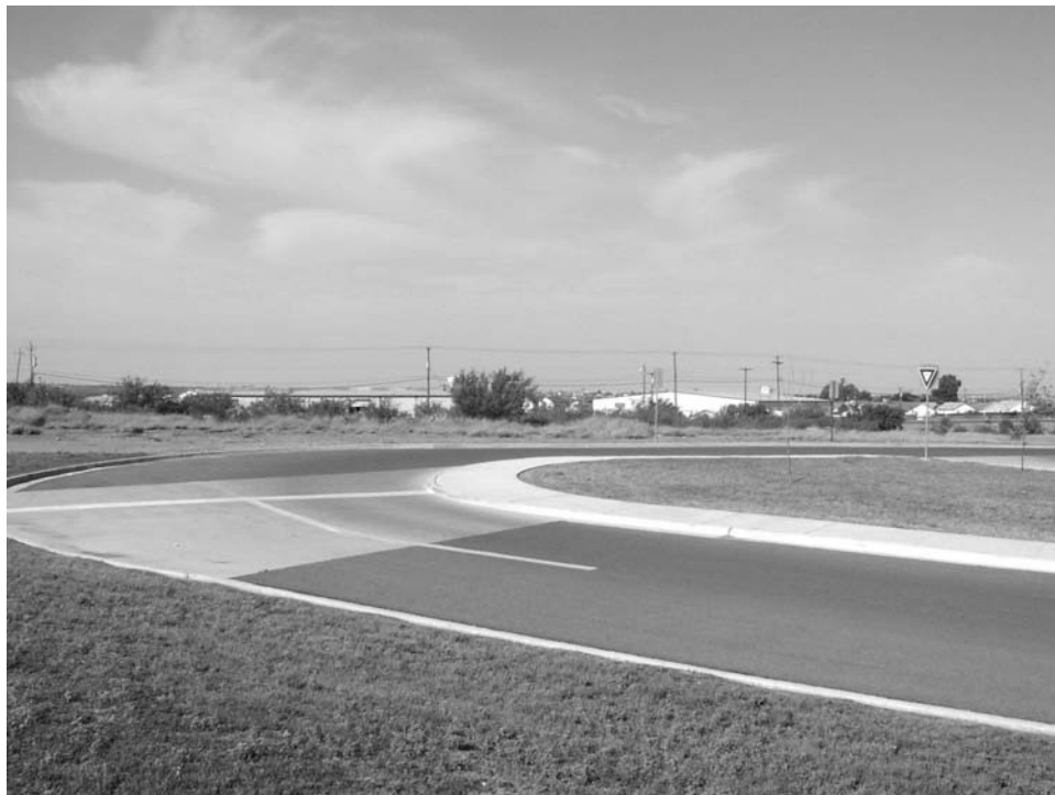
Figure 7-80. Driveway 4 (Facing Southwest).
