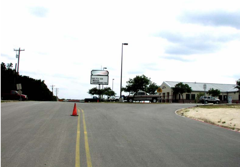
Figure 7-114. The Intermediate School Parent Drop-Off/Pick-Up Zone and Administration/Visitor Parking Lot (Facing South).
