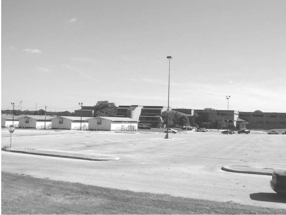
Figure 7-227. Student Parking Lots (Facing South).
