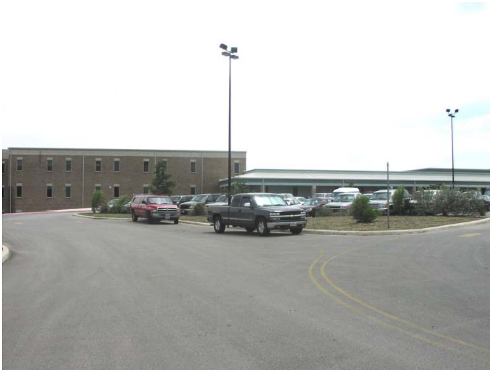
Figure 7-132. Administration/Visitor Parking Lot (Facing South).
