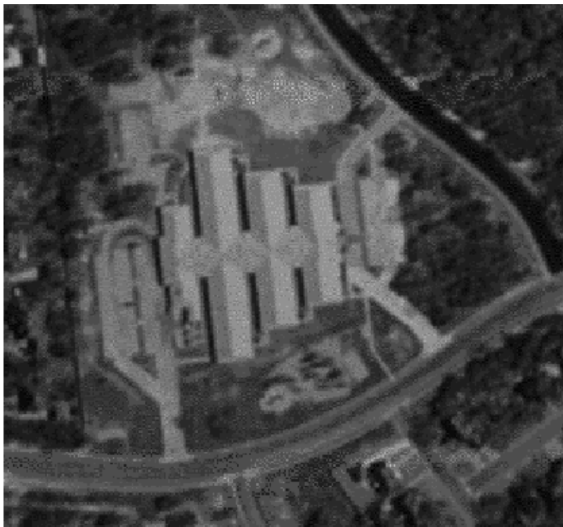
Figure 7-87. Aerial View of the Elementary School (47).
