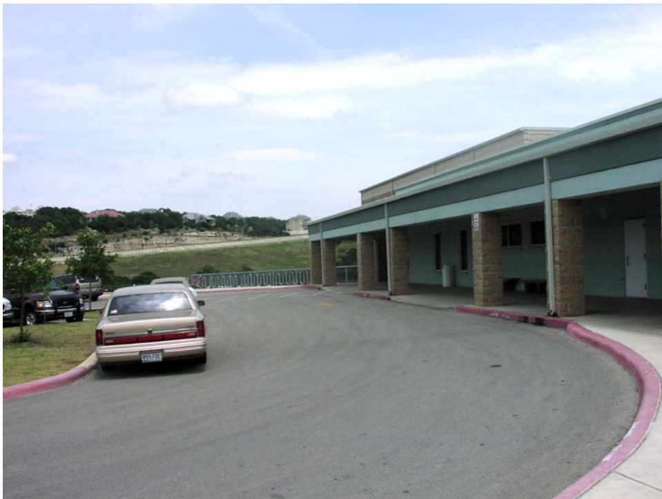
Figure 7-131. Parent Drop-Off/Pick-Up Zone (Facing Northeast).
