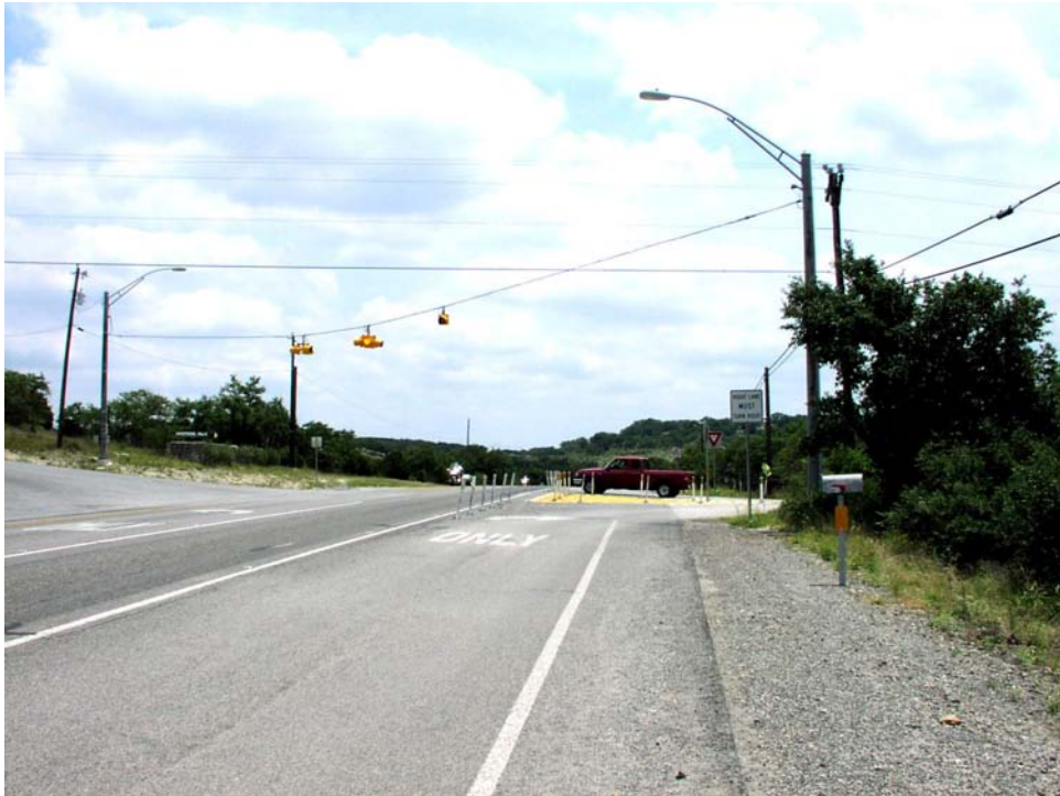
Figure 7-190. Driveway 1 (Facing East).
