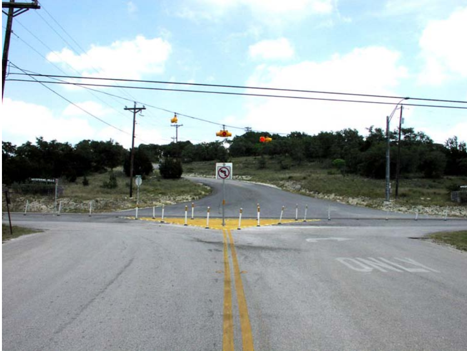
Figure 7-191. Driveway 1 (Facing North).
