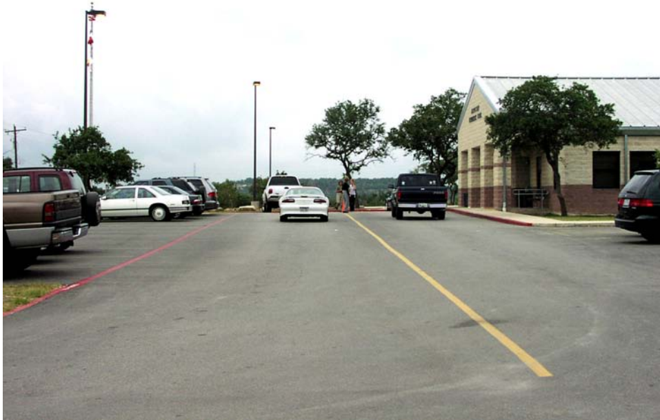
Figure 7-115. The Intermediate School Parent Drop-Off/Pick-Up Zone (Facing South).
