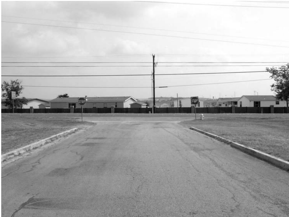
Figure 7-236. Driveway 5 (Facing Northeast).
