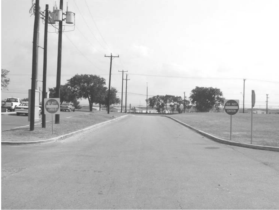
Figure 7-233 Driveway 4 (Facing Northeast).
