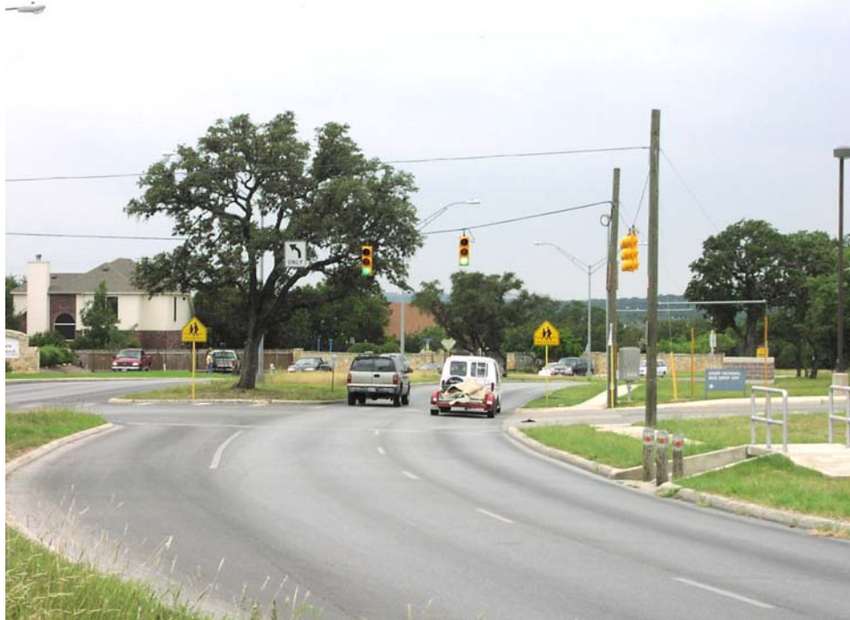
Figure 7-50. Driveway 2 (Facing Southwest).
