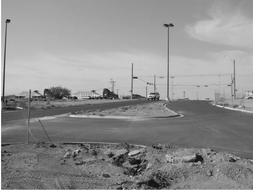
Figure 7-66. The Local Drive (Facing South).
