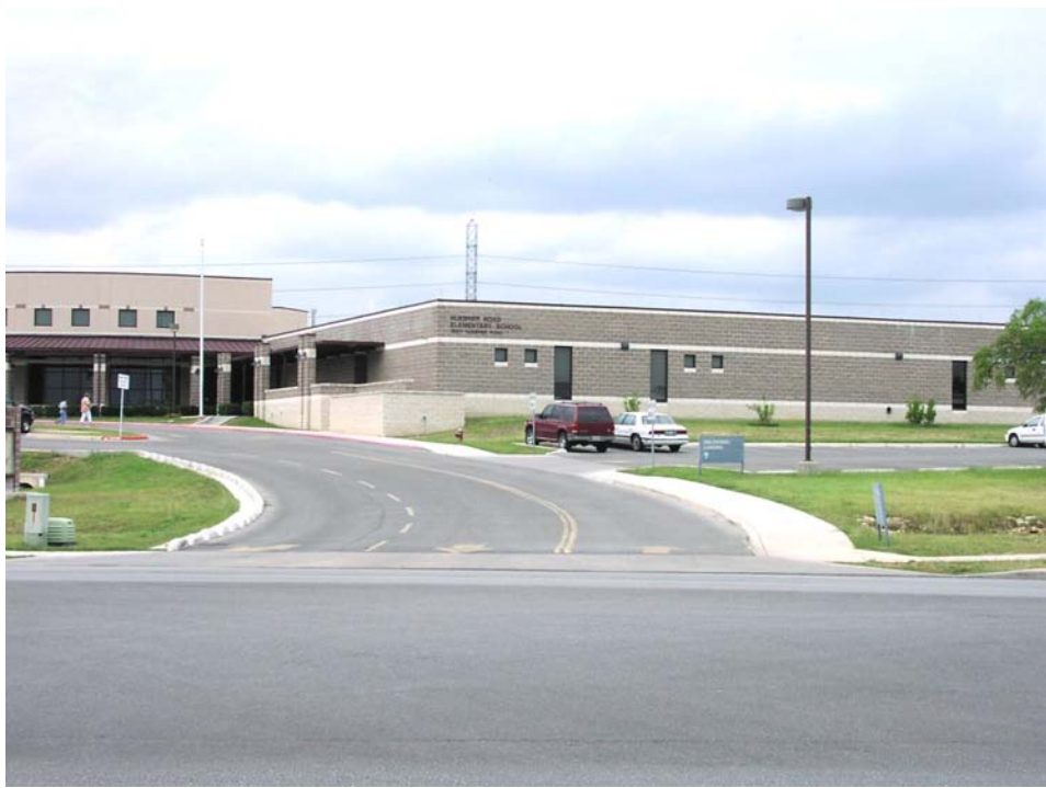
Figure 7-43. Driveway 1 (Facing North).
