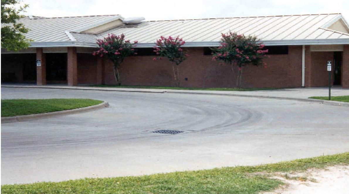
Figure 7-38. Curve in Bus Parking Lot.
