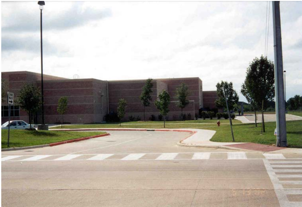
Figure 7-169. Entrance to the Bus and Visitor Parking Lot, Driveway 2.
