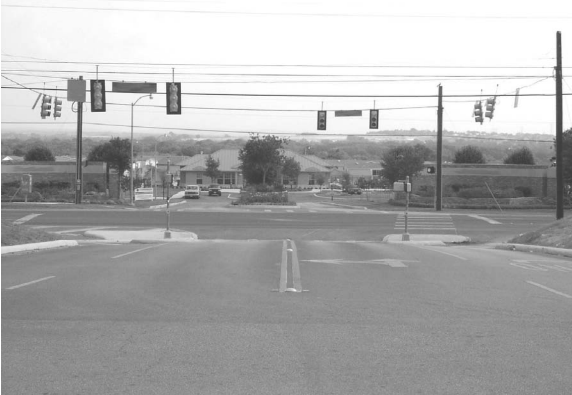
Figure 7-230. Driveway 3 (Facing Northeast).
